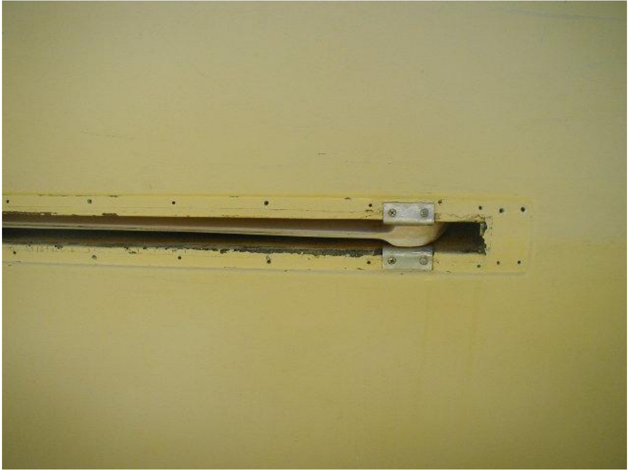
Cleaned up and ready to fill the holes.
