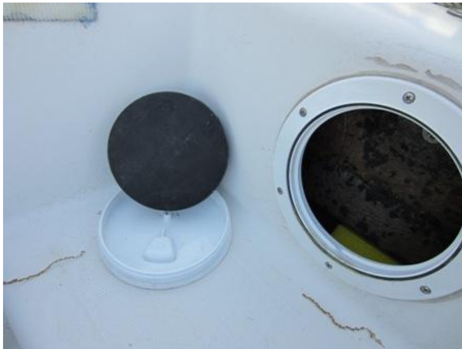
New inspection port compared to original black rubber plug.
